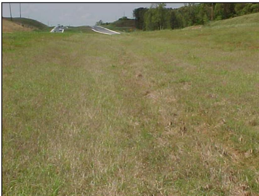
**Figure GS-1 Grass Swale in a Highway Median.**
