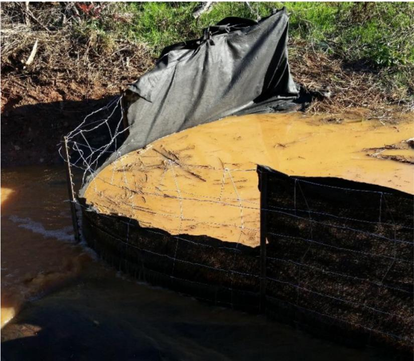
**Figure CD-7 Silt Fence Check Dam**
