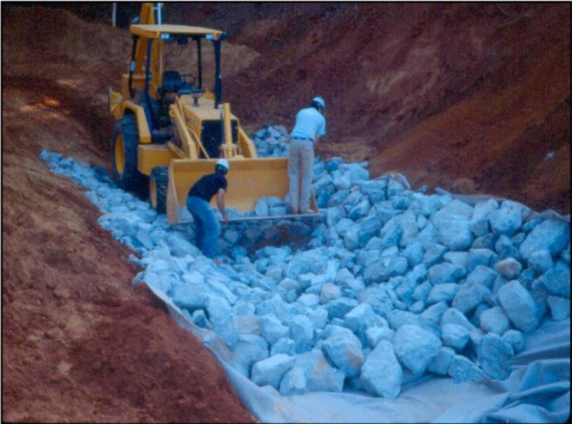
**Figure RS-1 Hand Placing Riprap.**
